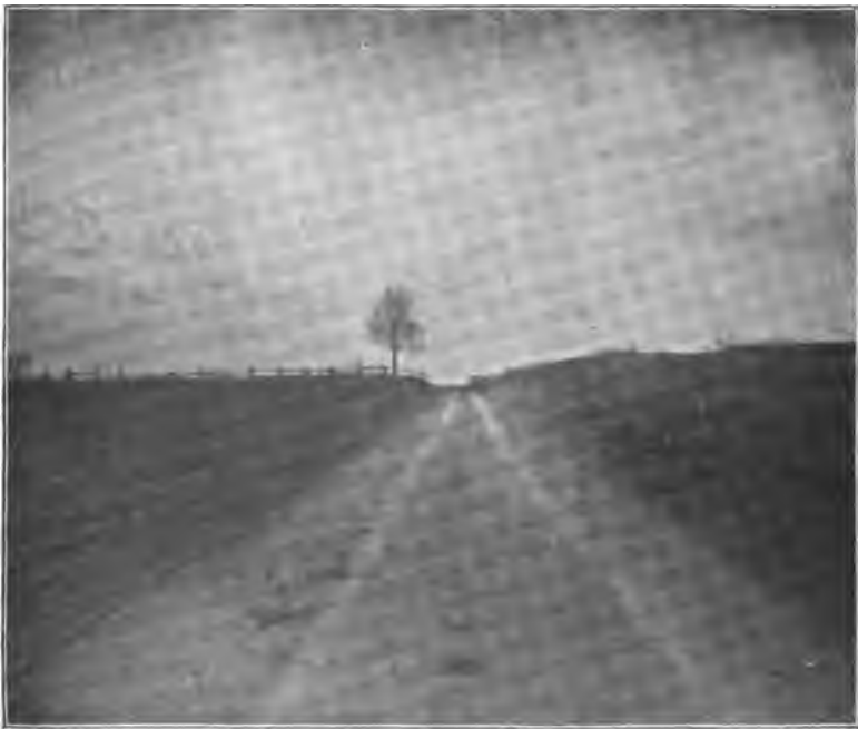
Stewartsville road, Warren Co., after improvement.
